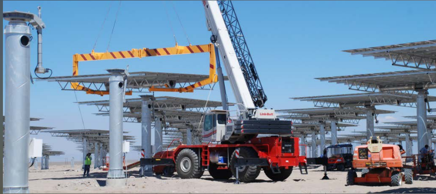
On-site heliostat assembly and installation
