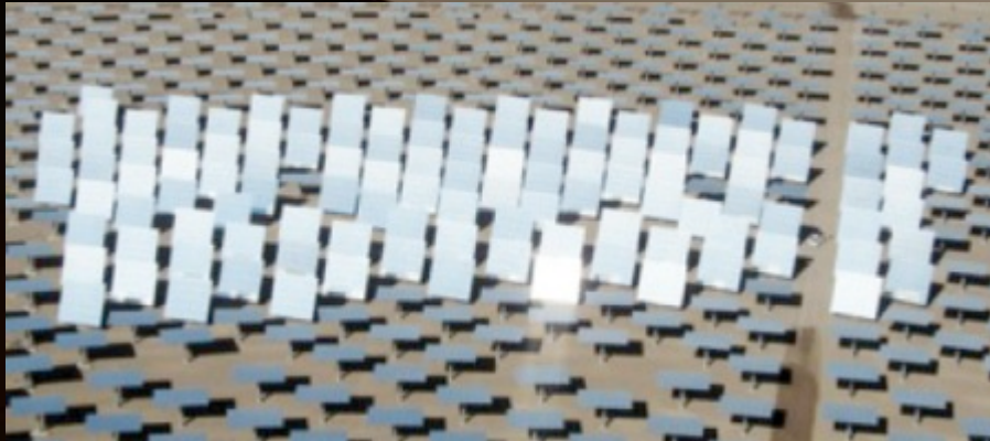
Dual axis tracking for optimal electricity production
