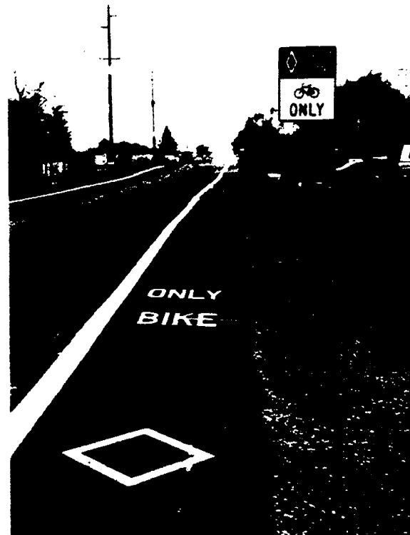
Bike lane sign and pavement markings
