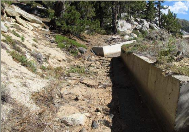
Marlette Dam Spillway
