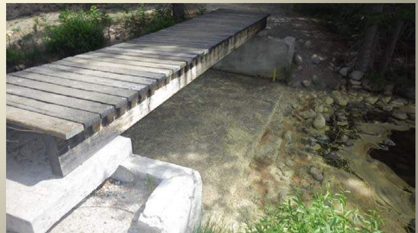
Hobart Dam Spillway
