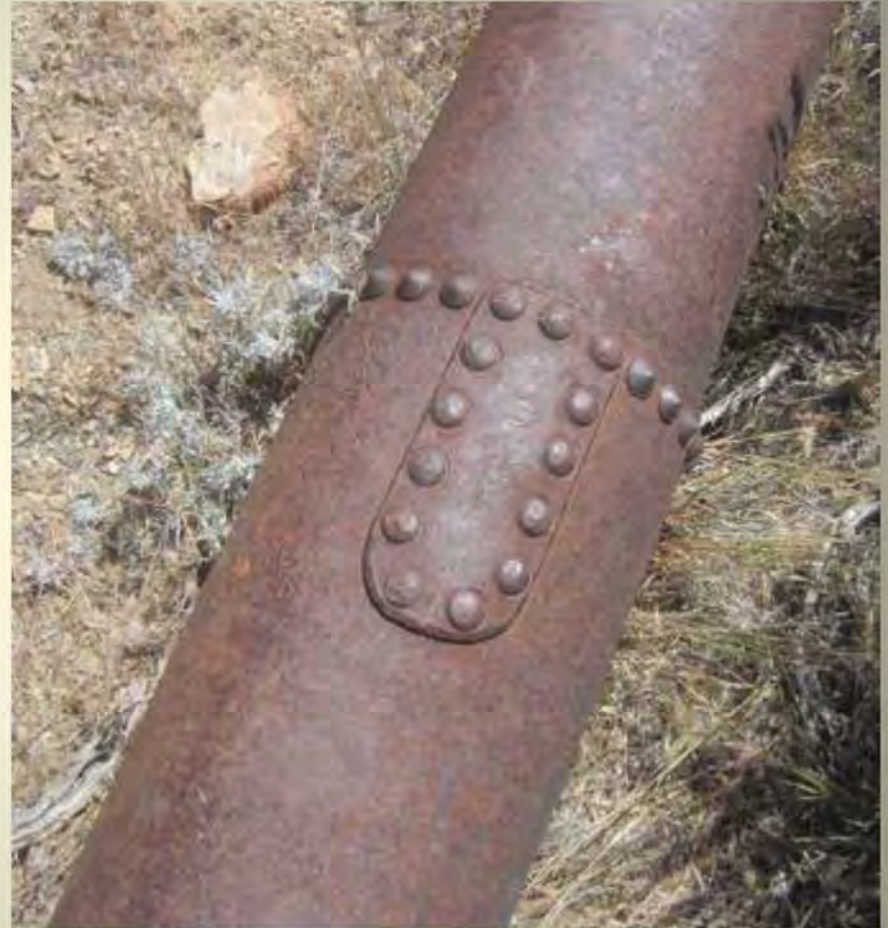
Pipeline-1 (riveted)
