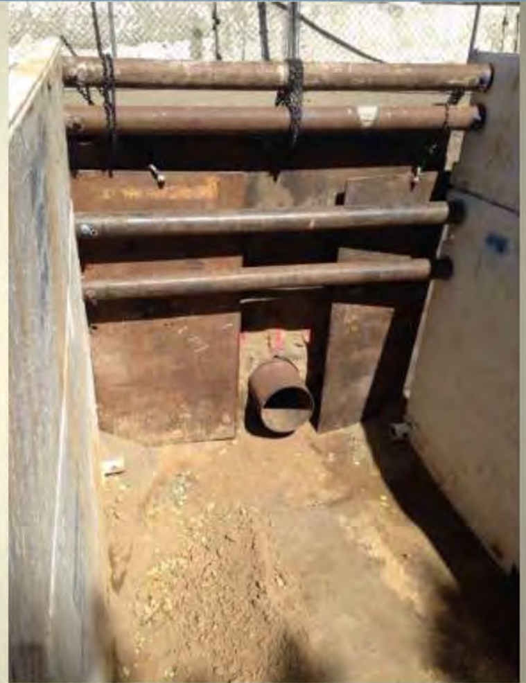
New Pipe Sleeve Installation Under I-580
