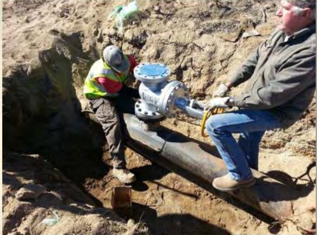
High Pressure Valve being Installed
