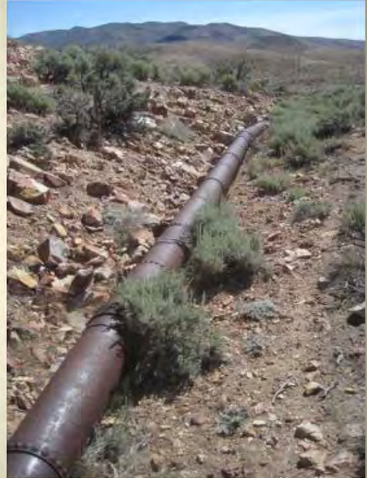
Pipeline-1 (Riveted Pipe)
