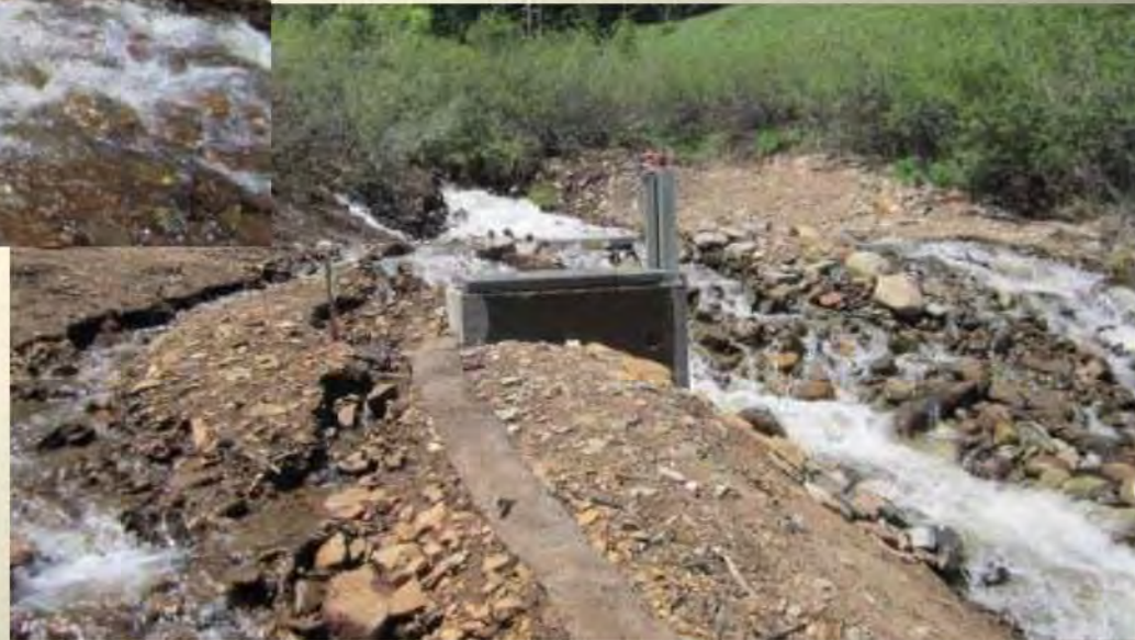
Sediment Trap Showing Runoff Bypassing Catchment
