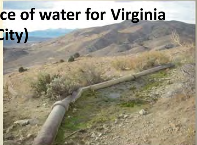
10" dia. lead joint pipe
