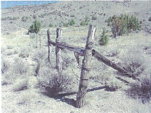
Collapsing exclosure fence near Dry Valley Spring (Washoe County) that is to be replaced.
