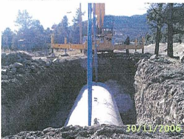
Above and below: Installation of dry hydrants in the Spring Valley / Double Springs chapter.
