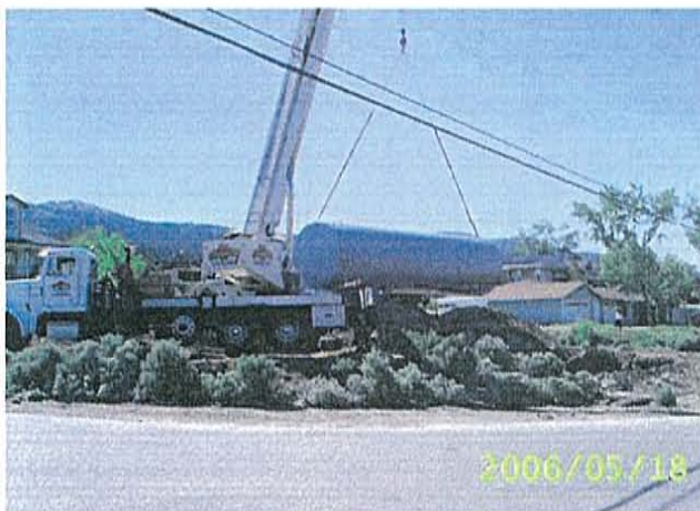
Above: Installation of a 10,000-gallon dry hydrant in the Pinion Hills neighborhood. Below: The nearly finished product, prior to landscaping.
