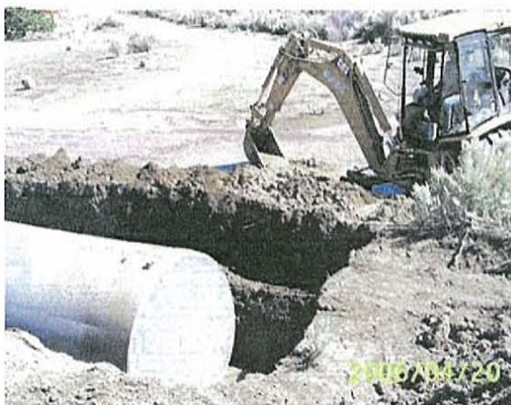
Above: Unloading the 10,000-gallon tank. Below: The tank is buried after being placed in the ground.
