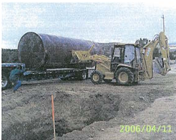
Above: Unloading the 10,000-gallon tank. Below: The tank is buried after being placed in the ground.
