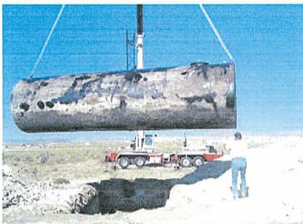
Left: a 10,000-gallon tank being installed in the community of Ryndon, Elko County, Nevada. Right: Mike McCarty, NVFSC project coordinator, shows the tank after installation. The pipe in the foreground is for firefighting equipment to draw water; the pipe in the background is an air vent and can also be used to fill the tank.
