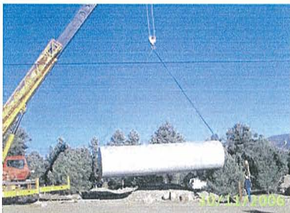
Above and below: Installation of dry hydrants in the Spring Valley / Double Springs chapter.
