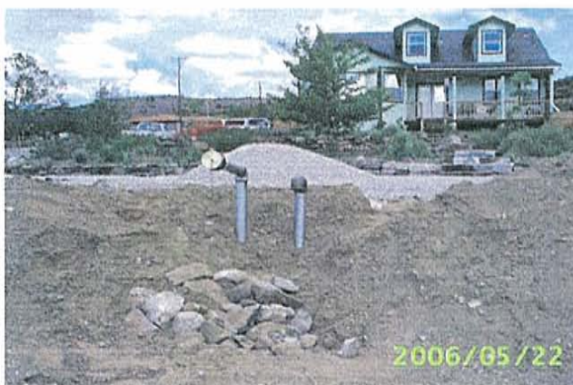
Above: Installation of a 10,000-gallon dry hydrant in the Pinion Hills neighborhood. Below: The nearly finished product, prior to landscaping.
