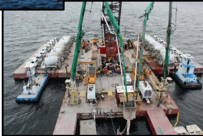
Tremi Concrete Pour: Concrete poured for 12 days, 24-hours a day.
