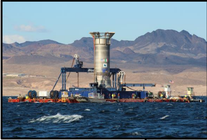
Intake Structure before it was lowered, being tugged out to final destination
