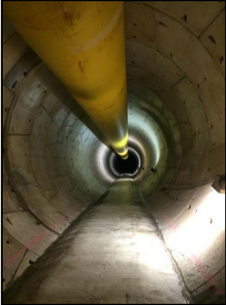
Intake tunnel, before it was put into service
