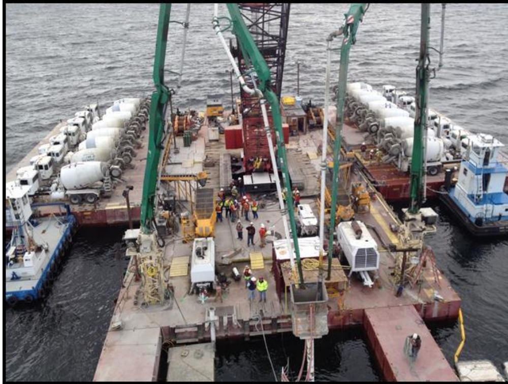
Cement trucks for intake structure placement
