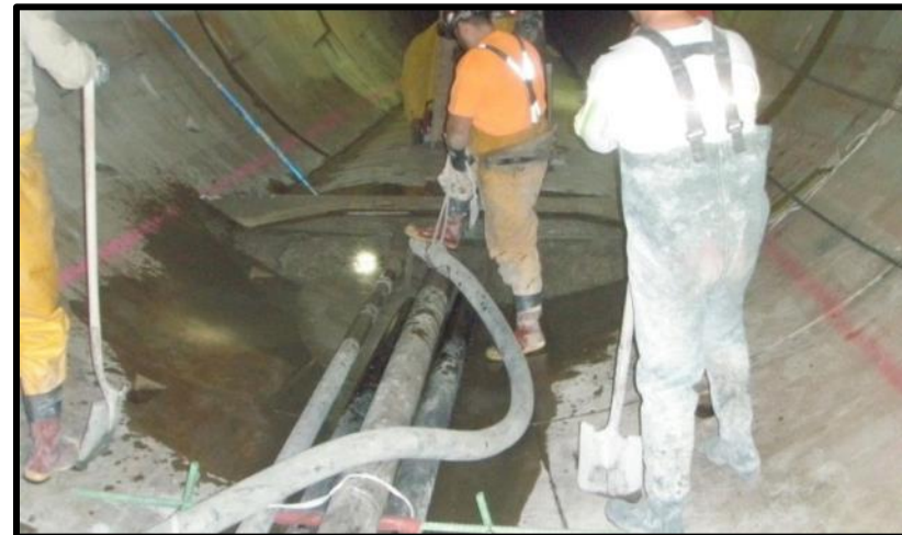
June 2015: Chemical Feed Line Installation
