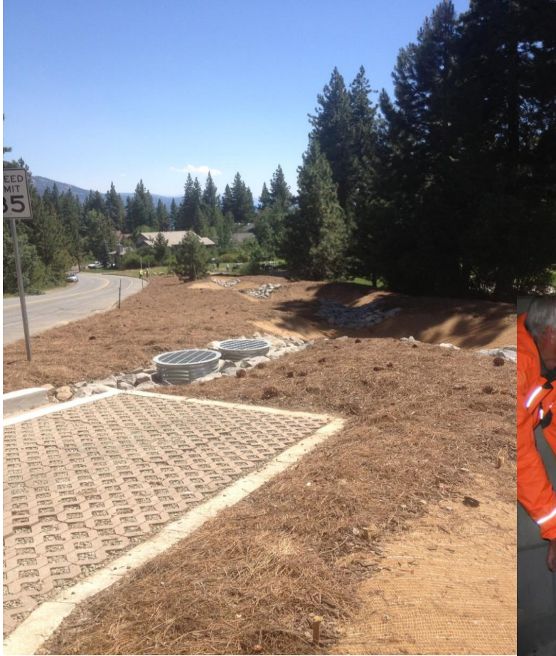
Newly constructed infiltration basin at Incline Village project.
