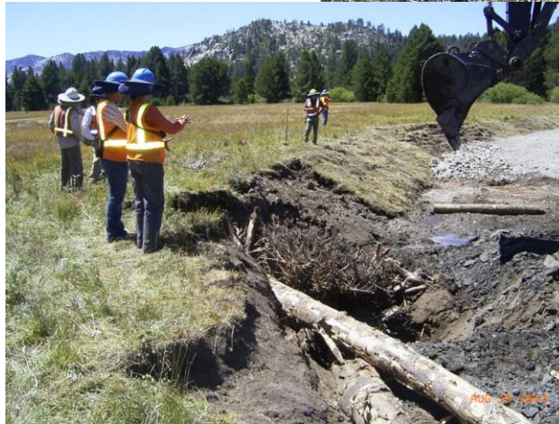
Logs are placed in the new channel of the Upper Truckee River during construction.
