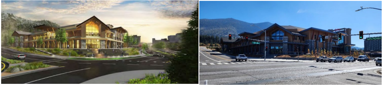
Source: TRPA Environmental Assessment Scoping Notice for the Tahoe South Events Center, 01.05.2018. Current photo taken on 10.27.2023
