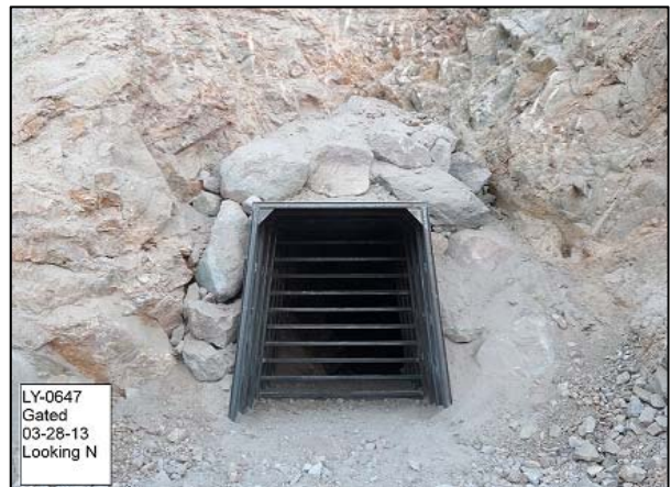
Example of a bat and bird compatible gate at the entrance of an abandoned mine site
