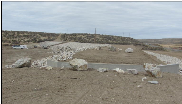
Jiggs Reservoir Dam after construction
