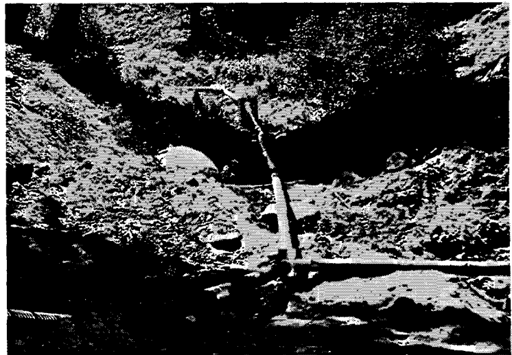
Fig. 33. Pipeline and catchment station installed in 1968 near east portal of tunnel.
