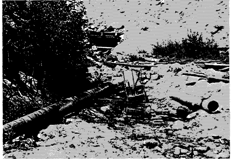
Fig. 32. East portal of tunnel, 1968, showing installation of catchment weir to capture water flow.
