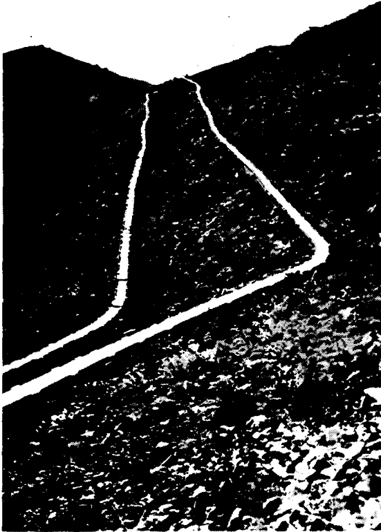
Fig. 5. Flumes in the Virginia Range: Five-Mile Reservoir to Virginia City, c. 1877.
