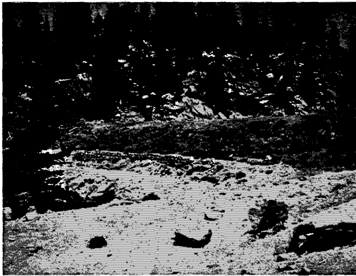
Fig. 15. Southwest face of Marlette Dam showing level of old dam and additional structure above placed by Curtiss-Wright, 1968.
