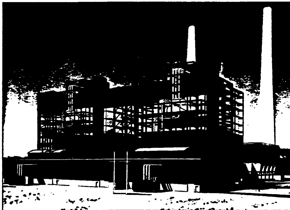
250 megawatt coal-fired units
